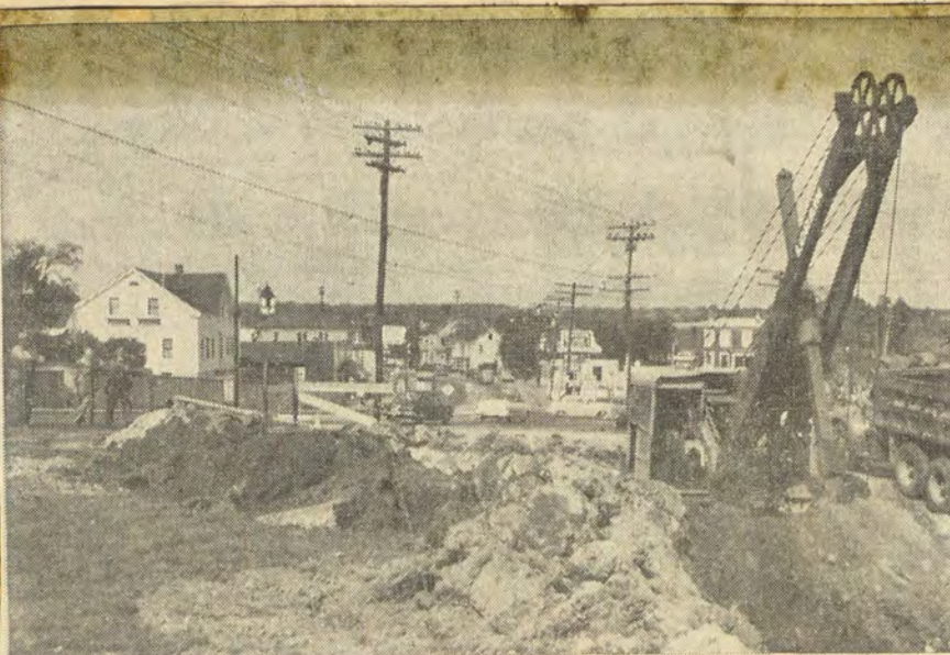
Power shovel takes big bites out of ground at site on Main Street, Arctic, where three-way municipal building will be erected by Frank W. Johnson & Son construction firm. Shovel is digging at approximate site where old police station stood. —(Times Photo)
