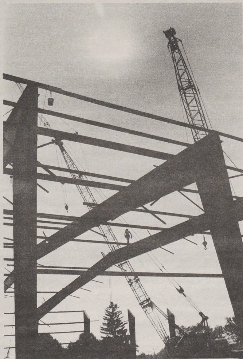
MORE THAN 320 TONS of steel supply the framework for the College's new recreation center. Work continues toward a late January opening. (What's News Photo by Gordon E. Rowley)
