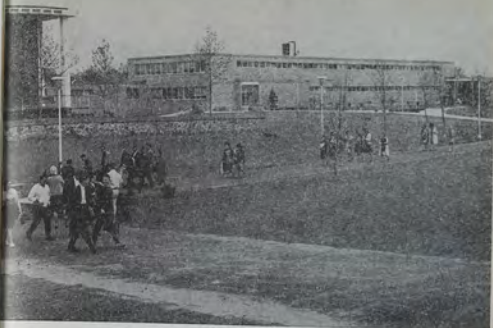
John Clarke Science Building
