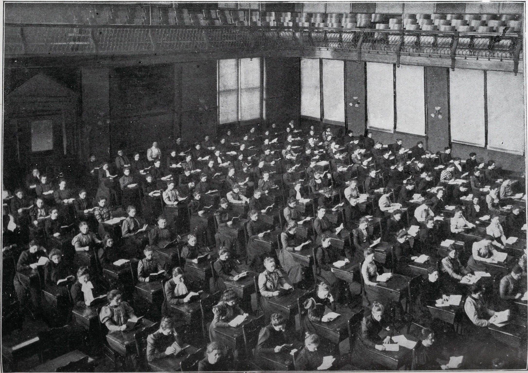
THE ASSEMBLY HALL.
