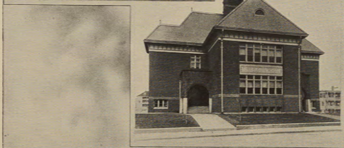
Lincoln Avenue School, West Barrington
