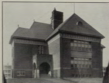
Garfield Street School, Central Falls
