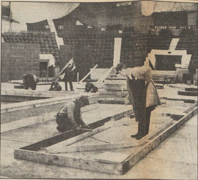
This View of Huge Arena, Showing William E. Brigham, Artistic Floor Director, Standing in Foreground, Gives a Glimpse of Features of the Exhibition Opening in the Middle of the Week. Mr. Brigham is Superintending the Construction of Frames for the Parterre Gardens, Which Will Surround the Pool for Aquatic Plants, a Corner of Which is Shown at the Left. Also at the Left Can Be Seen a Portion of the 12-Foot Fence Which Will Entirely Surround the Floor and Be Made to Resemble a Stone Wall. The Motif of This Year's Flower Show, Sponsored by the Associated Garden Clubs of Rhode Island, is a Formal Italian Garden, of Which the Pool, and a Cascade at the East End of the Hall Are to Be Features. Opening Wednesday, the Show Will Continue Through Next Sunday.
