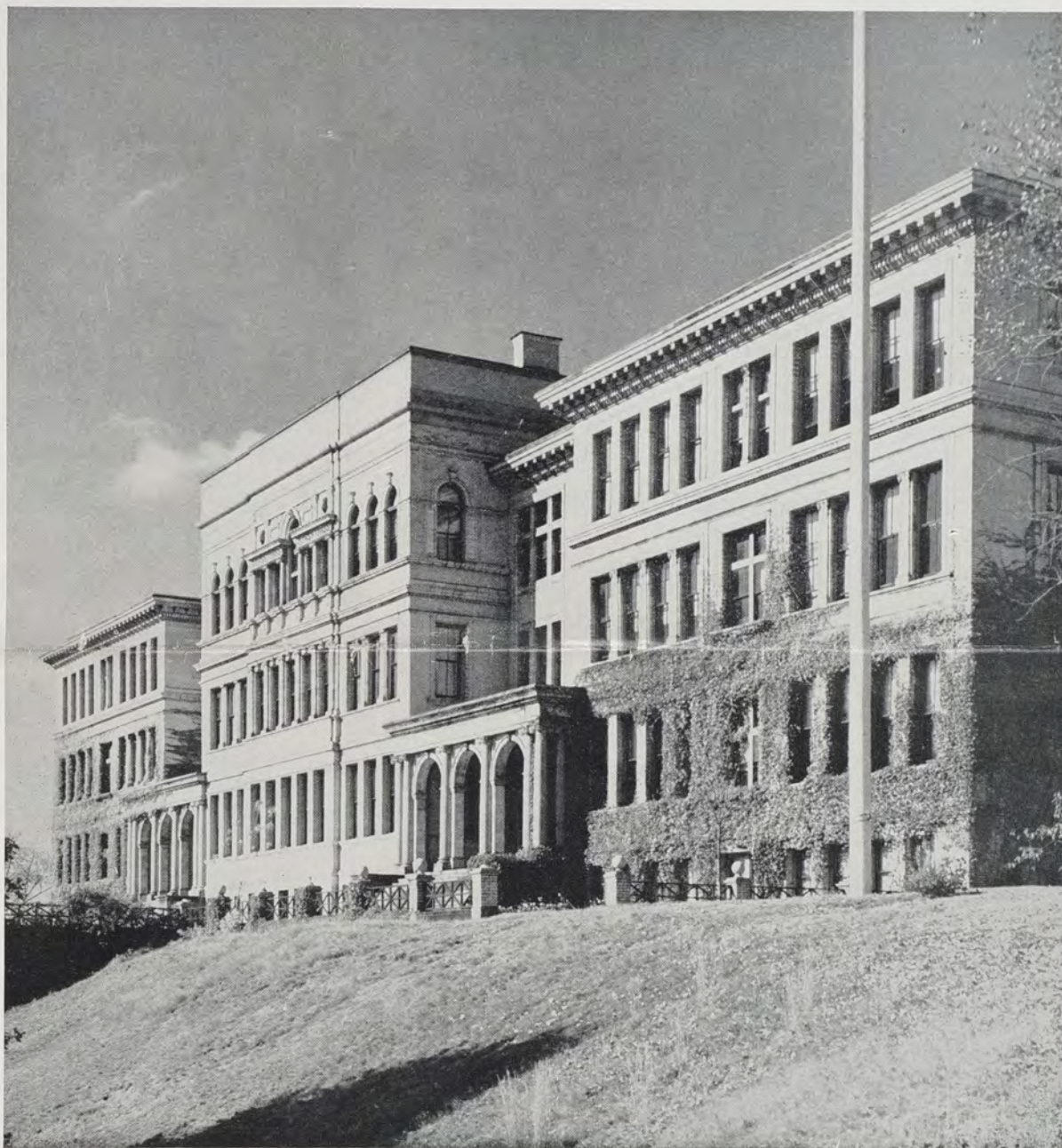
To this old building we dedicate this memorial issue.
