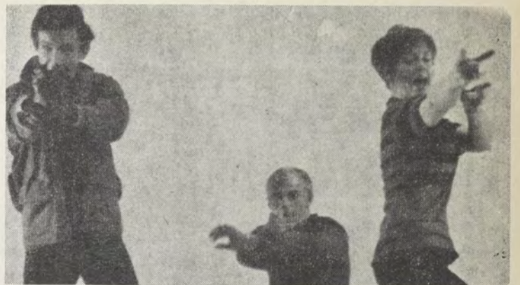
Radicals attacking the administration building
