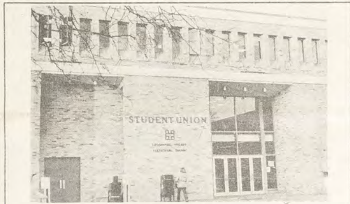
Student Union Roof Under Repair
