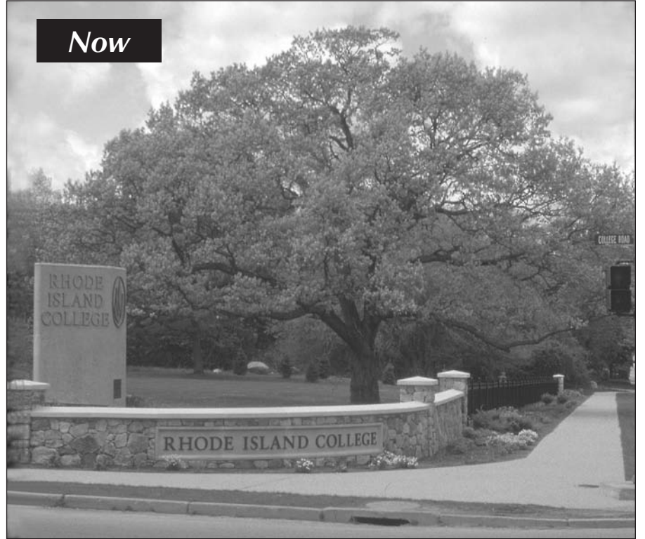
AND NOW: This is the greatly enhanced Mt. Pleasant entrance, including the 1964 monument as well as a new masonry wall, iron fencing and landscaping. The improvements were made as part of this year's Sesquicentennial celebration. In the background is the Sesquicentennial Oak, still standing, despite partial destruction from hurricane remnant winds on Sept. 11, 2002.
