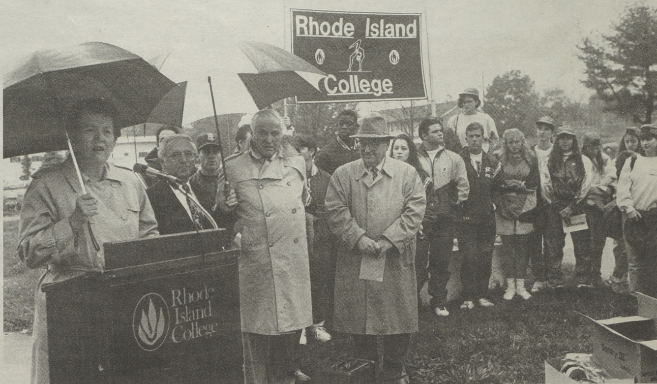
RAINY SKIES, BRIGHT SPIRITS: Vice President Lenore DeLucia (far left) gives some history about the RIC campus and its buildings before officially breaking ground during ceremonies marking the beginning of the construction of the College's new $8.8 million health, physical education and athletic complex. To her left is President John Nazarian, Governor Bruce Sundlun, Higher Education Commissioner Americo Petrocelli, and a host of student-athletics. (What's News Photo by Gordon E. Rowley)
