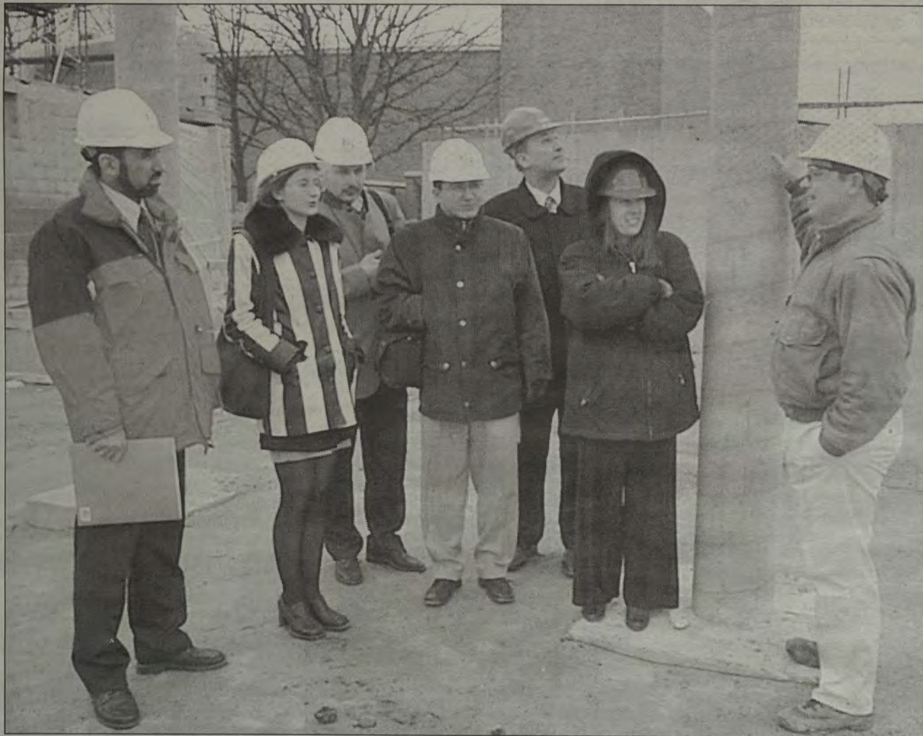
RUSSIAN VISITORS: Four construction contractors from the former Soviet Union and their interpreters toured the new performing arts classroom facility under construction next to Roberts Hall on March 11. Their visit to Rhode Island was sponsored by area Rotary Clubs. Standing in what will soon be the lobby of the new theater are (l to r) Arsen Khatchaturov, Maria Ozhekh, Alexander Gvozdkov, Alexander Ananyev, Mikhail Beliaev, Masha Entchevitch, and Jack Kowal, site superintendent for Hodess Building Company. (What's News Photo by Gordon E. Rowley)
